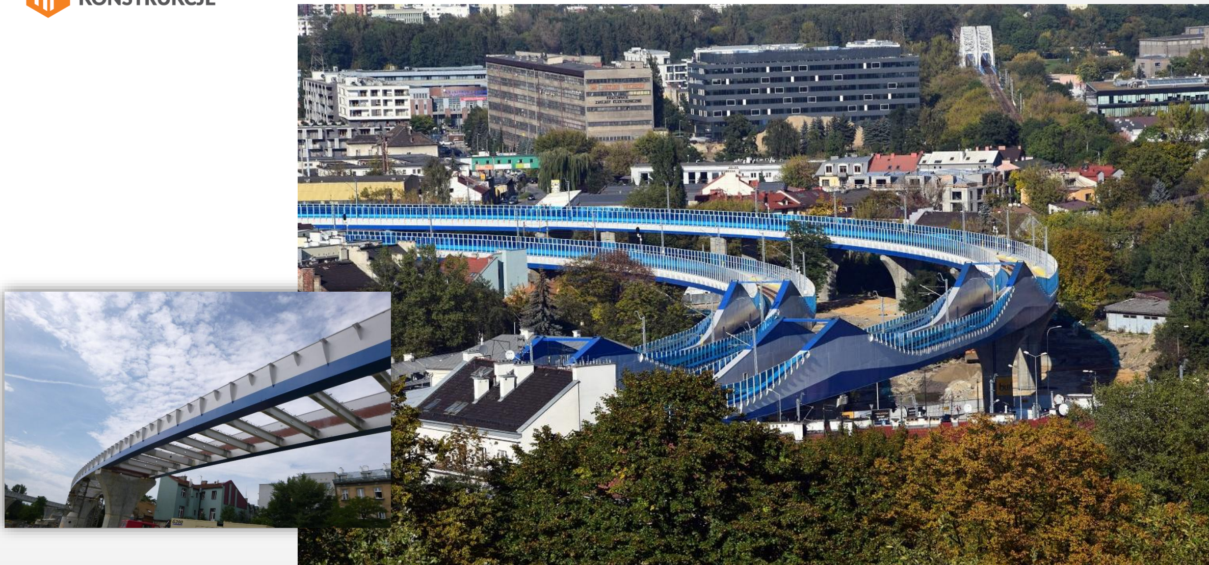
Estakada ES-1 KRAKÓW
